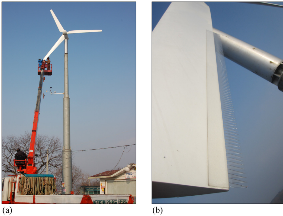
Fig. 2 – Photos of (a) the 10kW wind turbine and (b) attached trailing edge serration
